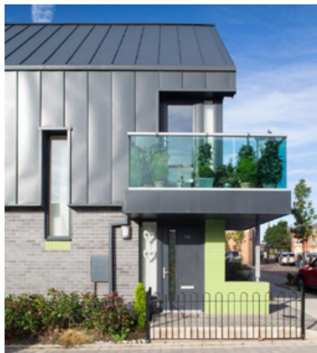
Catnic® Urban (formerly Colorcoat Urban®) standing seam steel system, is a lightweight, strong and versatile alternative to traditional building materials that is seven times lighter than standard roof tiles.
