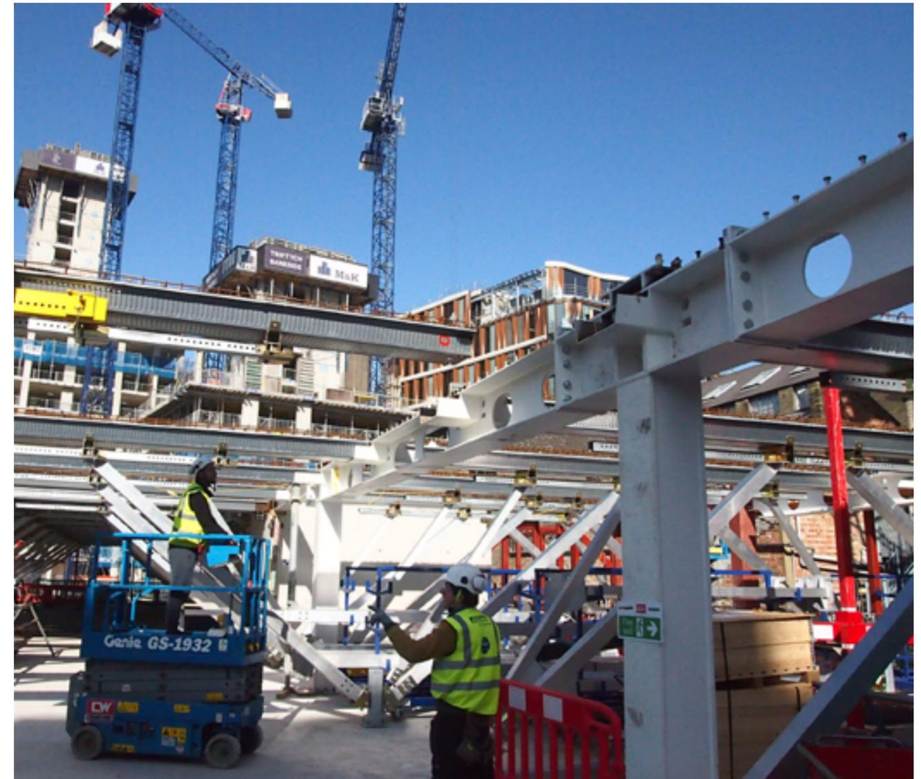
The Forge in London, the UK's first net zero carbon commercial building, contains Tata Steel's ComFlor® beam, specifically designed for a pioneering construction technique: a platform approach to design for manufacture and assembly known as P-DfMA.
