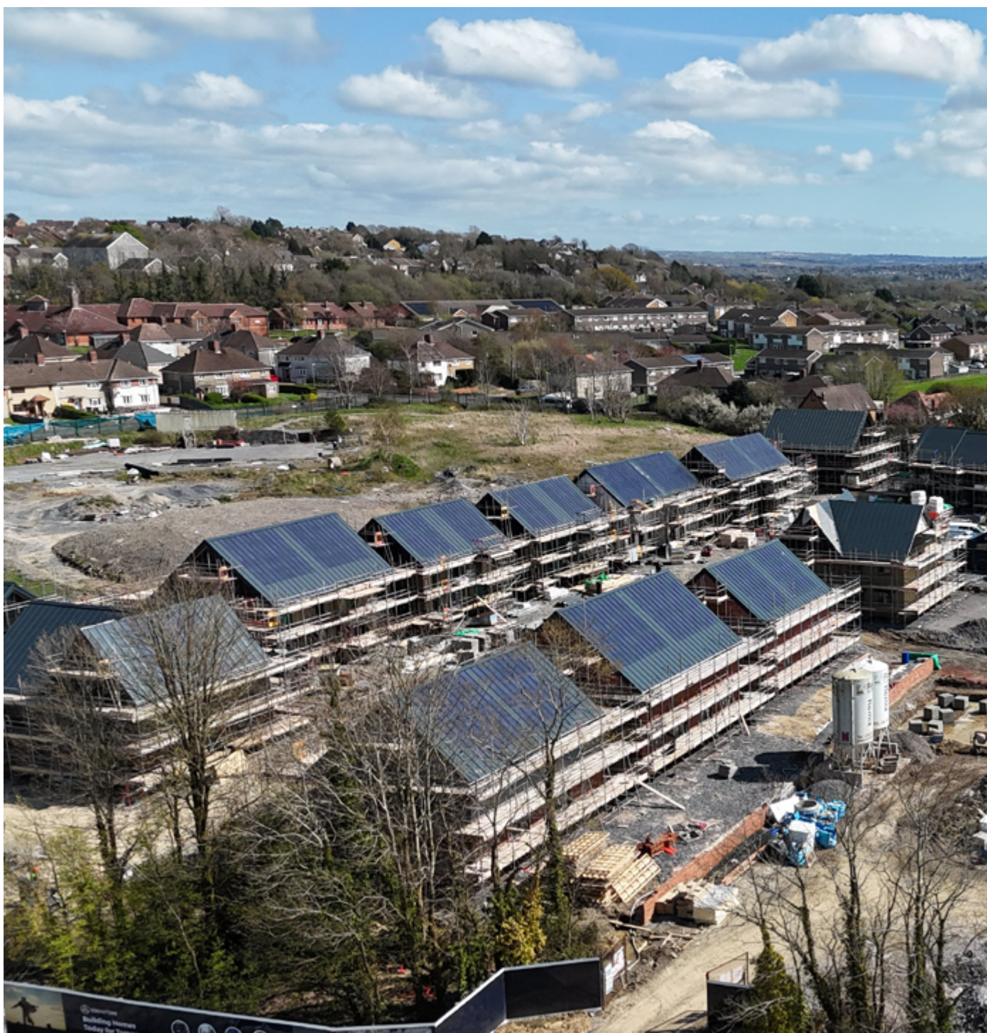
At Pemberton coastal social housing development, SolarSeam is being installed across 70 homes.
