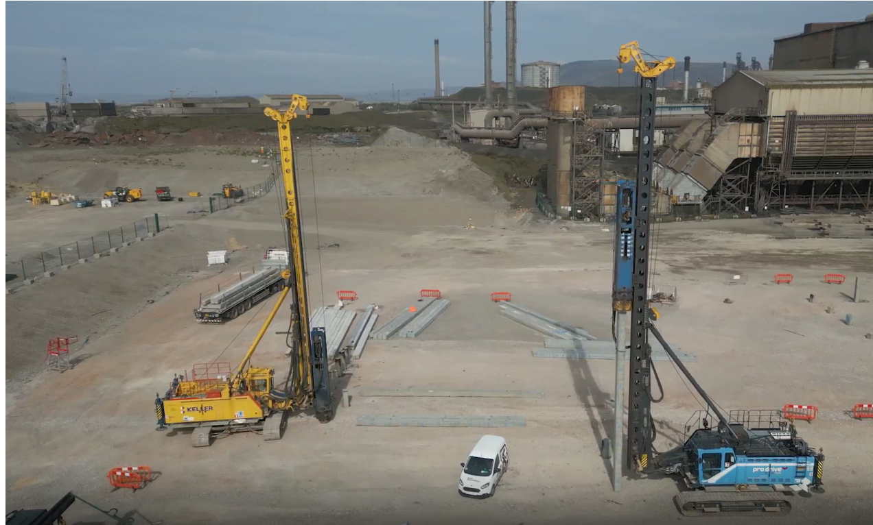
Solid foundations – piling rigs go to work at Port Talbot
