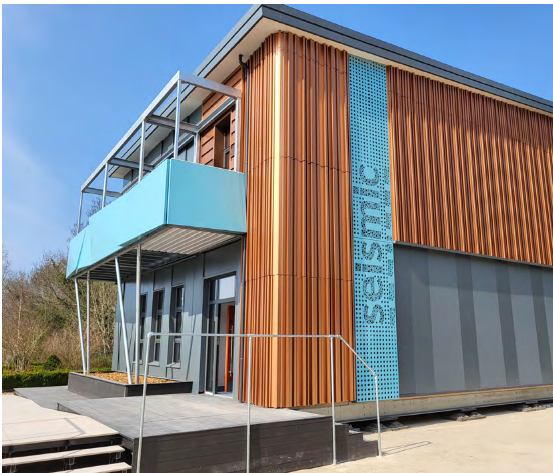
The Seismic demonstrator building.
